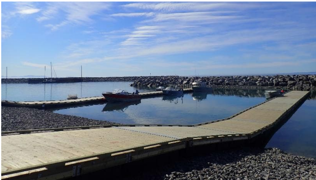
Figure 6-3 Pond Inlet Floating Docks
