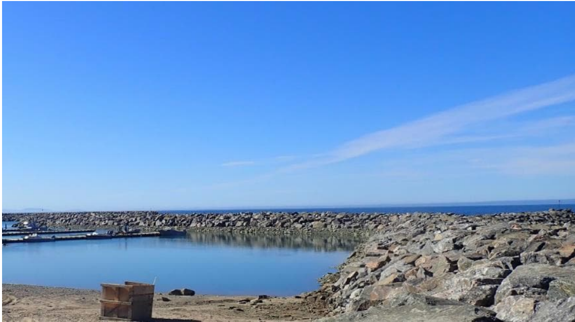
Figure 6-1 Breakwater, Pond Inlet
