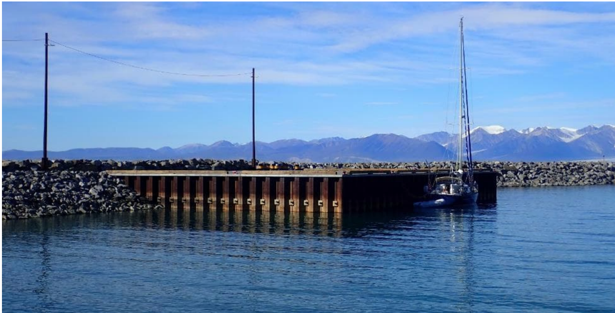
Figure 6-4 Fixed Dock, Pond Inlet
