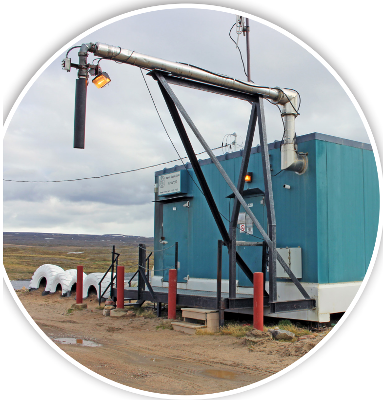
Pond Inlet Water Treatment Plant
