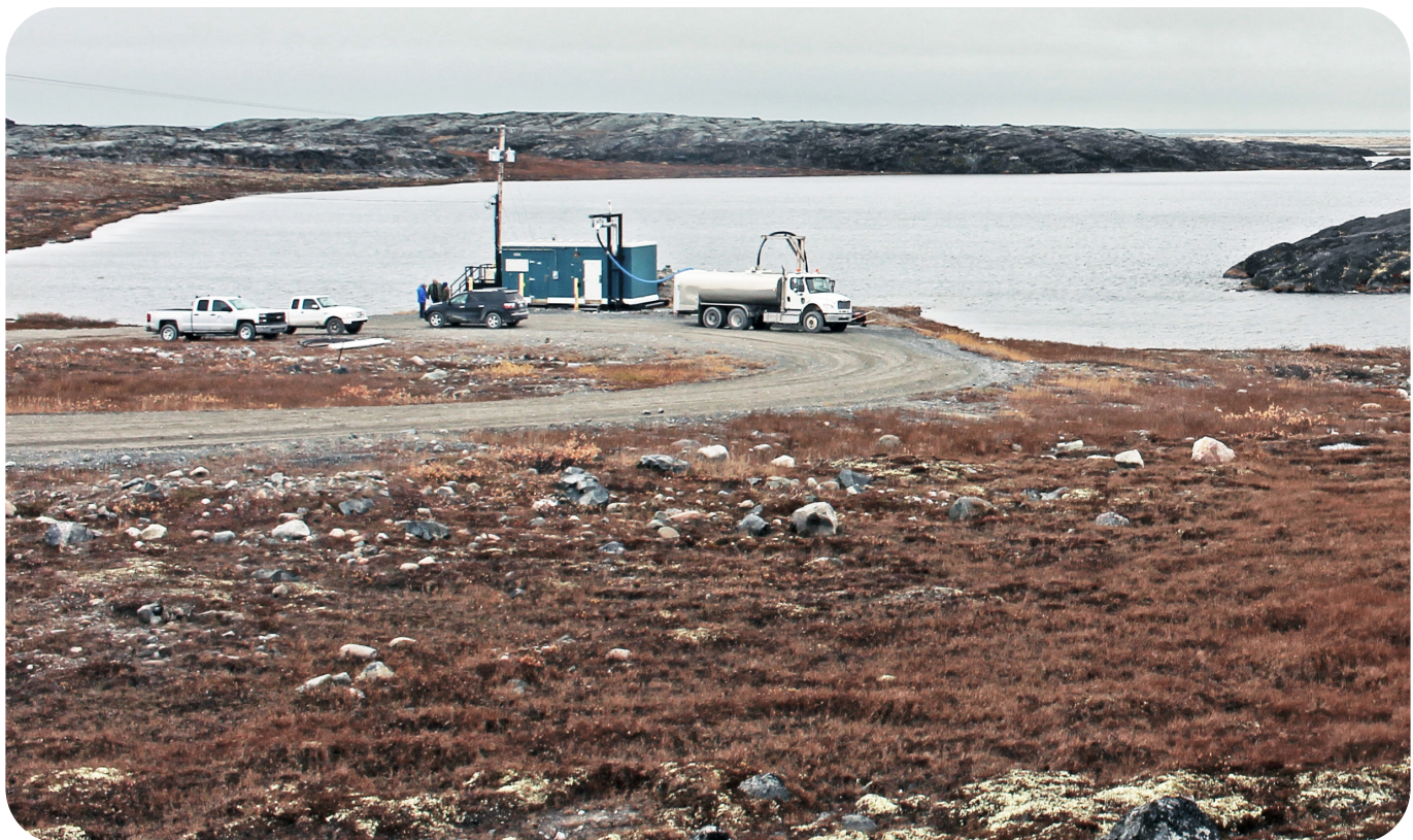
Whale Cove Water Treatment Plant
