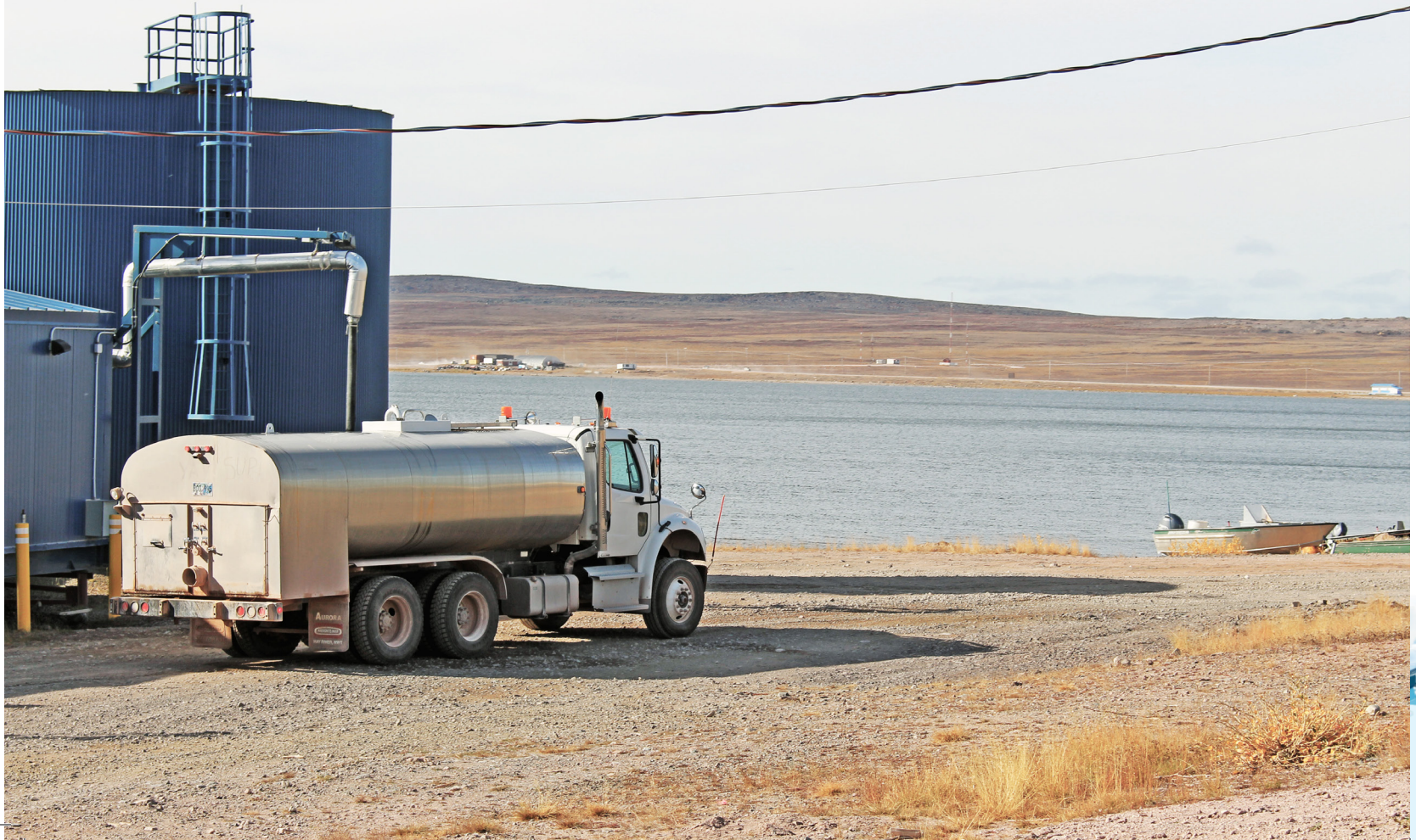
Baker Lake Truckfill
